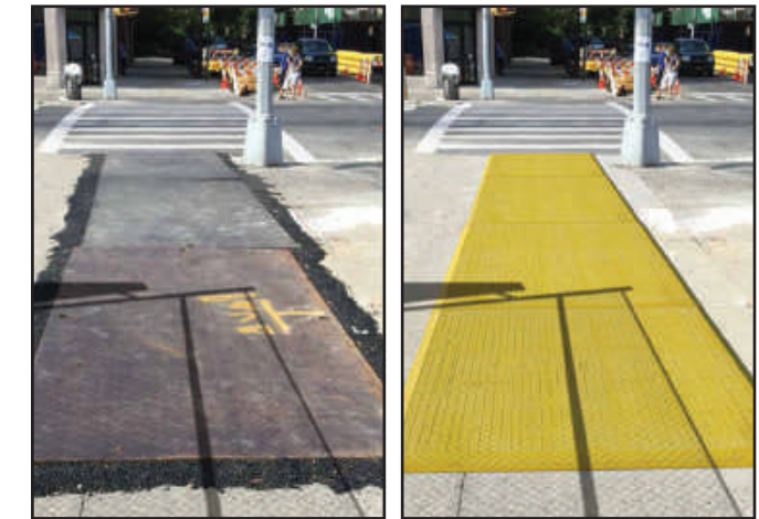
Steel Plates with Cold Patch
