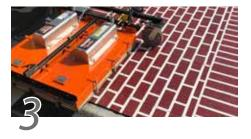
Heat material until sufficiently bonded to the surface
